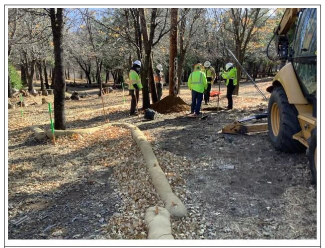
**Photo 1:** A crew was observed digging a direct bury pole hole at Pole P40211 (C 440) within clearly delineated work limits in accordance with MM BIO-1.
