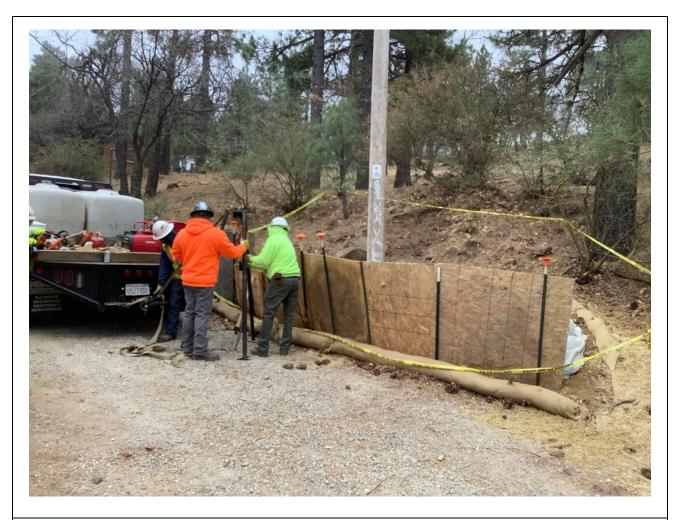
**Photo 6:** A crew was observed maintaining plywood erosion control BMPs at Pole P40430 (C 440) to contain spoils within the work area in accordance with APM HYD-09, the ECP, and the SWPPP (MM HYD-1, MM BIO-7).
