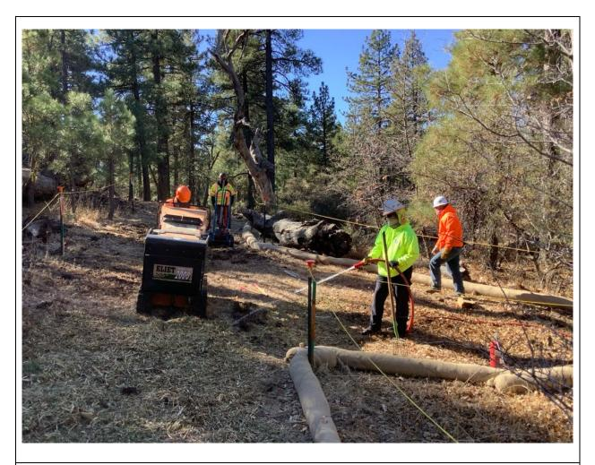
**Photo 4:** A crew was observed chipping along the underground alignment near Pole P40289 (C 440). A full set of fire tools was observed within 50 feet of the activity, at least 100 gallons of water with pump and hose were observed on site, and the area was wet down to prevent ignitions in accordance with the CFPPP for chipping on NFS land with a PAL C.
